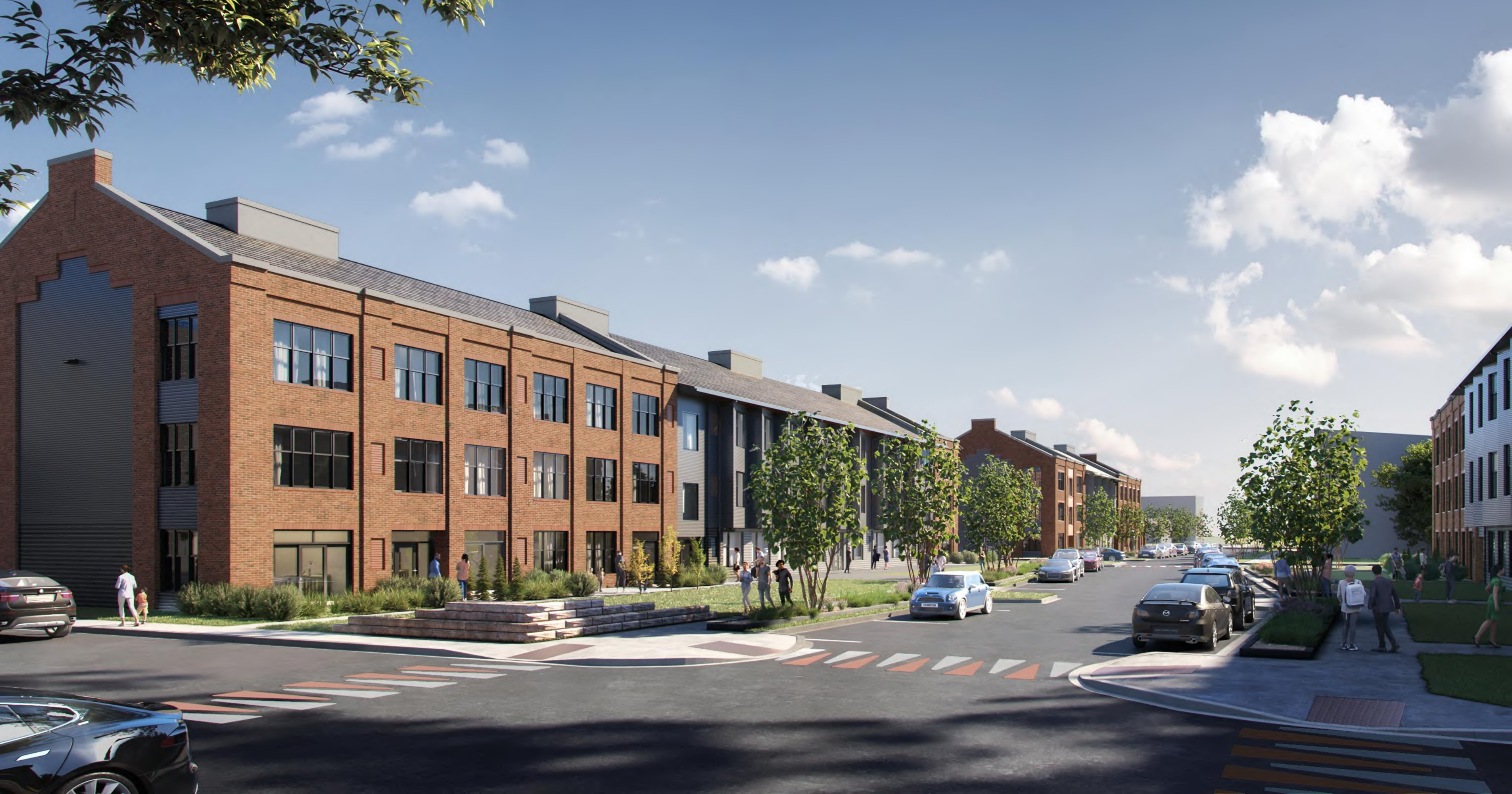
New Street and Park View looking North
