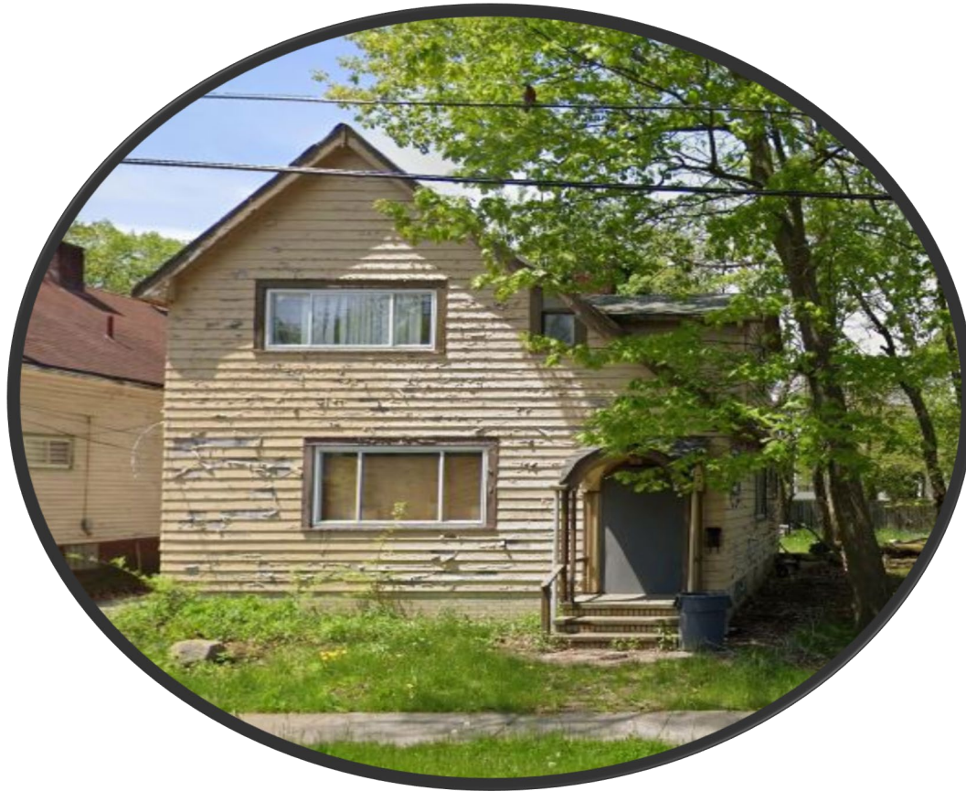
Proposed Demolition of 2868 E. 114 th St.
